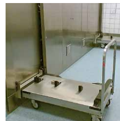
Docking a transfer trolley on the sterilizer
